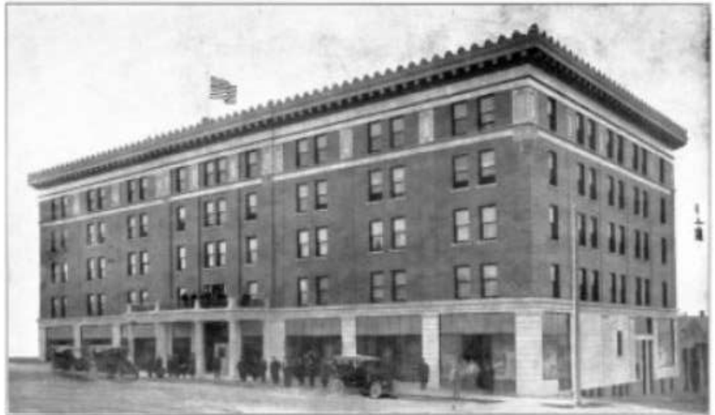
NEW MC CHARLES HOTEL, ABSOLUTELY FIRE-PROOF. 200 ROOMS, 24 BATHS, AMERICAN PLAN, $2.00 TO $3.00 PER DAY. FERRIS, N. D.
