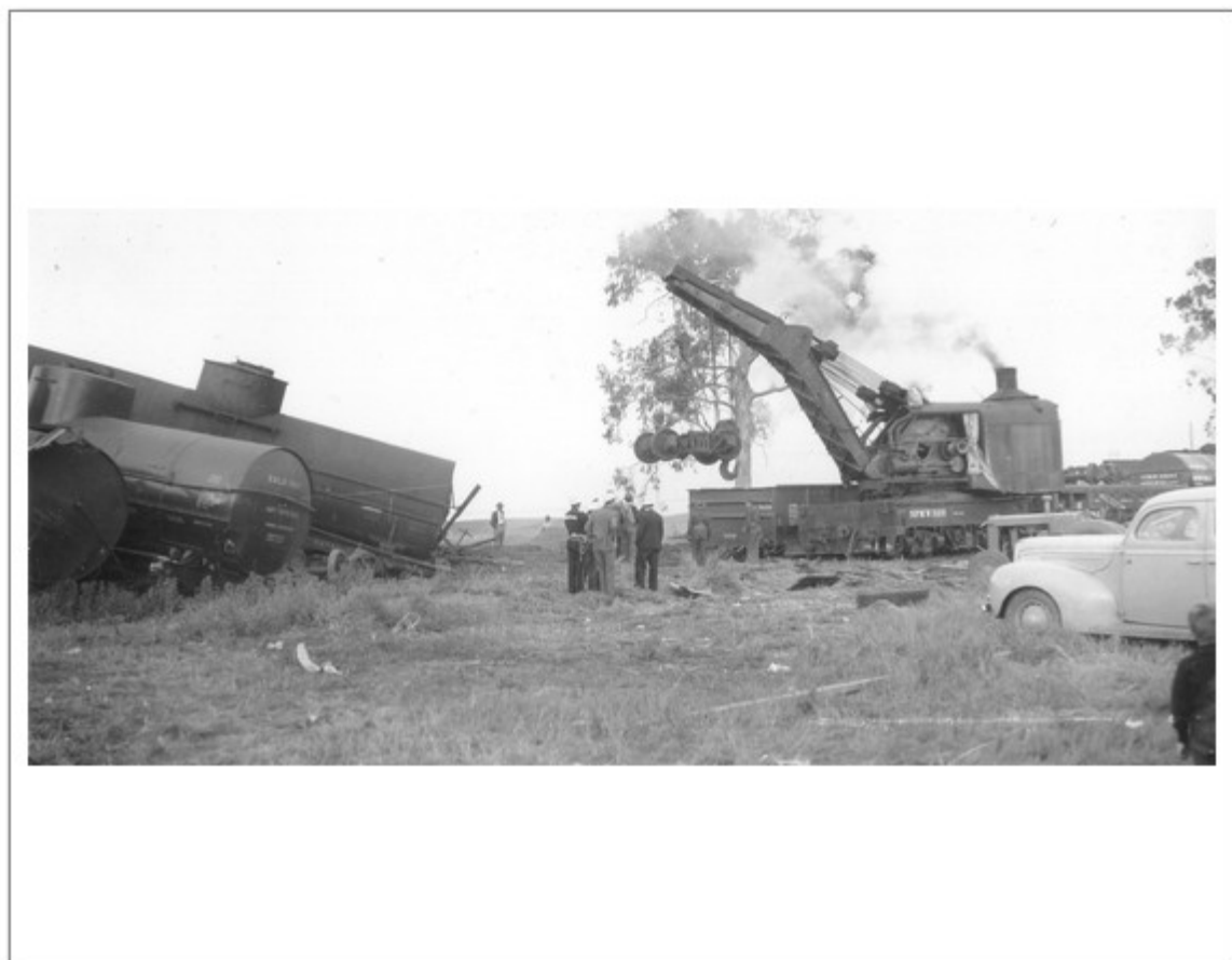
246-Crane clearing the train wreckage from the tracks
