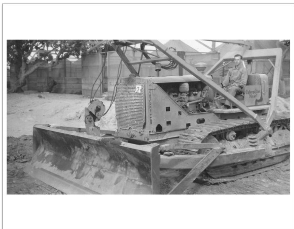
242-Private Tunnis Zwiép driving bulldozer
