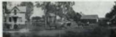
RESIDENCE AND FARM BUILDINGS OF I. W. WHITNEY.
