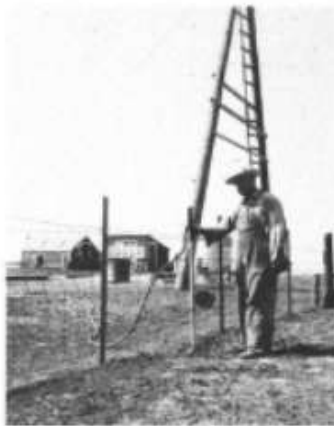
John Fitzgerald & First Water Hydrant-1946
