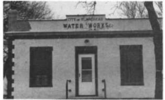
Flandreau Water Works
