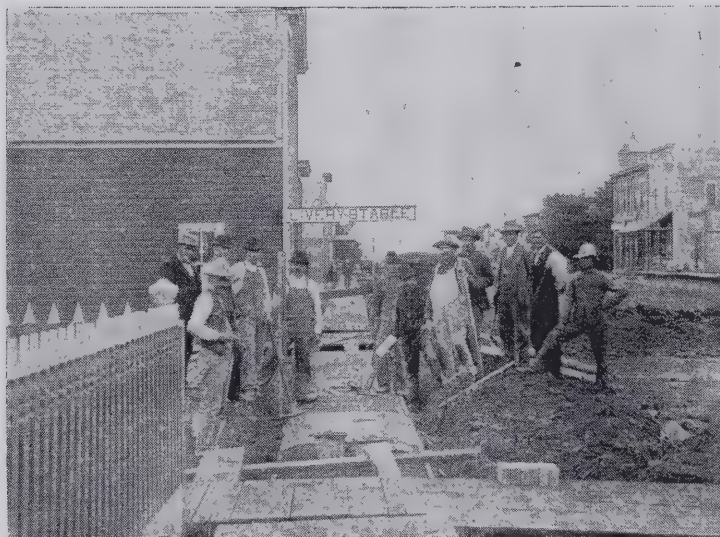
REPLACING BOARD SIDEWALKS WITH CEMENT WALKS
