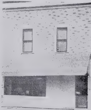
FIRST BUILDING IN FREEMAN on present Schamber corner which is today the Laber Meat Market.
